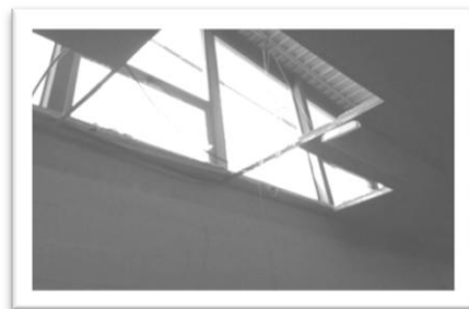
Window access from the roof
